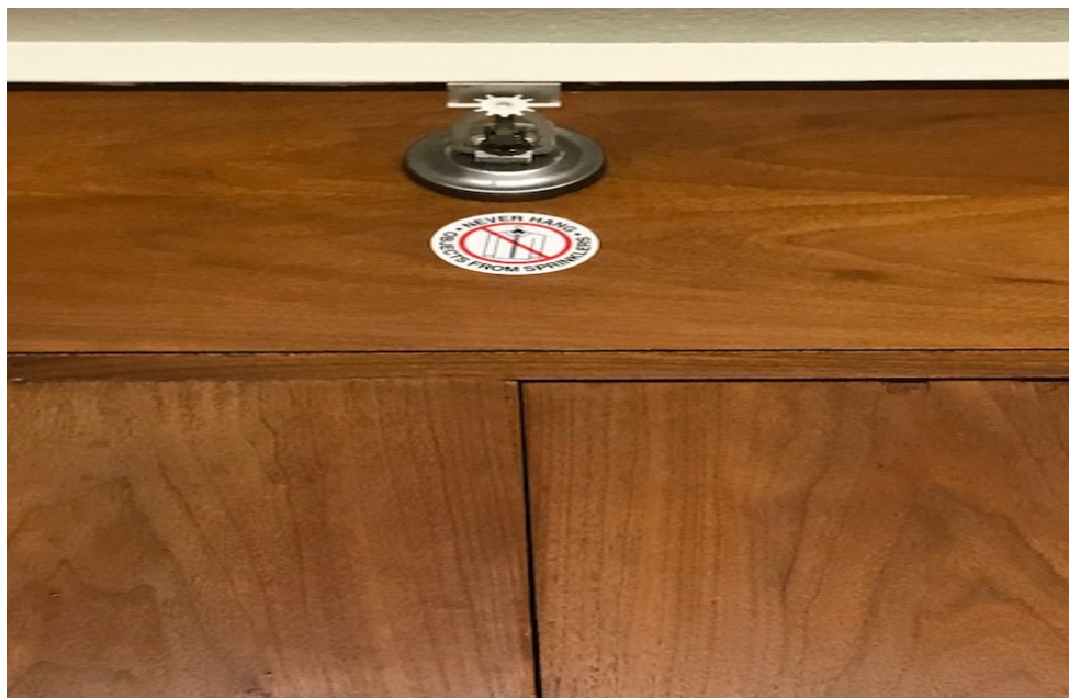
Figure 1 Rhoads Hall - On Closet
