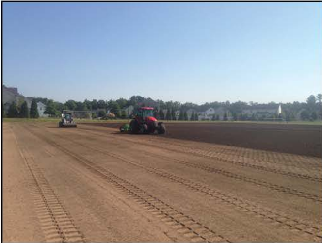
Image 6 - Blecavate (Reverse Tine Tilling) (1)
