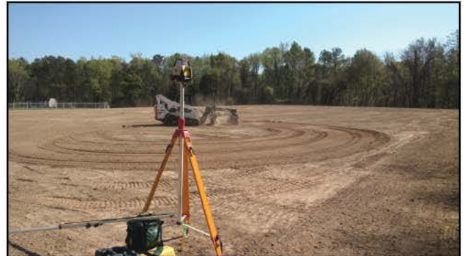
Image 8 - Laser Guided Hydraulic Blading (1)
