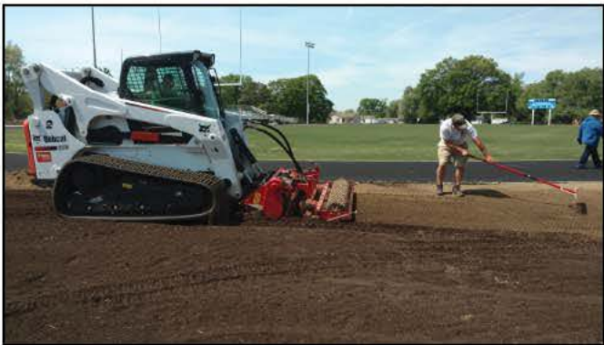
Image 7 - Blecavate (Reverse Tine Tilling) (2)
